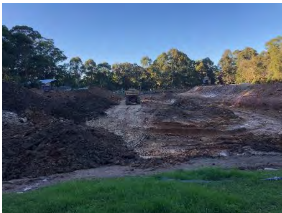
Works as at 30 June 2023
