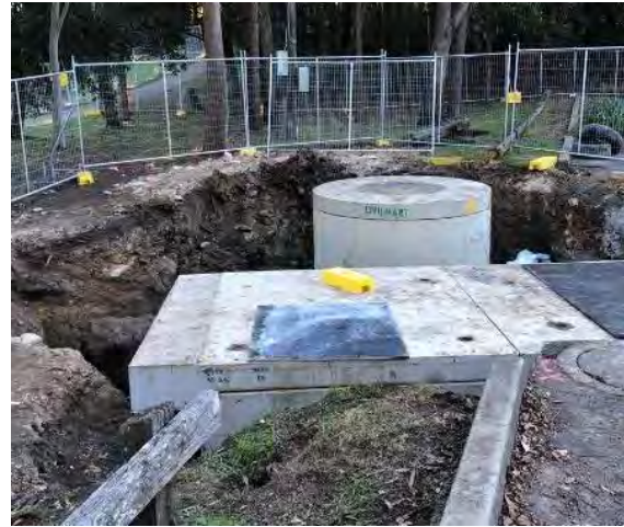
The gross pollution trap and diversion to underground detention but what about the water flow from the hill above the field?
