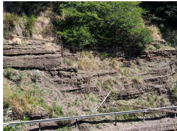
Mittagong Formation type locality – cutting of the Gib Tunnel, Mittagong
