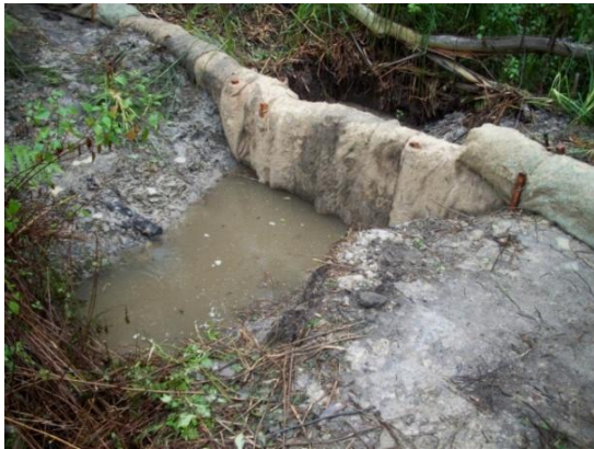
Figure 4. Phillip Road outlet stabilisation and treatment (complete and operating)
