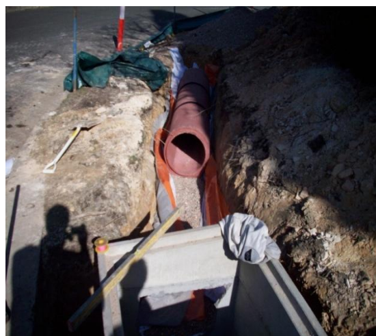
Figure 2. Milburn Place stormwater filter pipe
