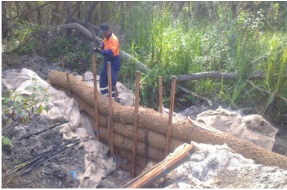
Figure 3. Phillip Road outlet stabilisation and treatment (during construction)
