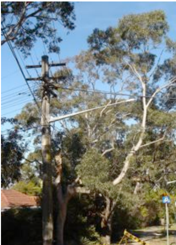
A damaged eucalypt
