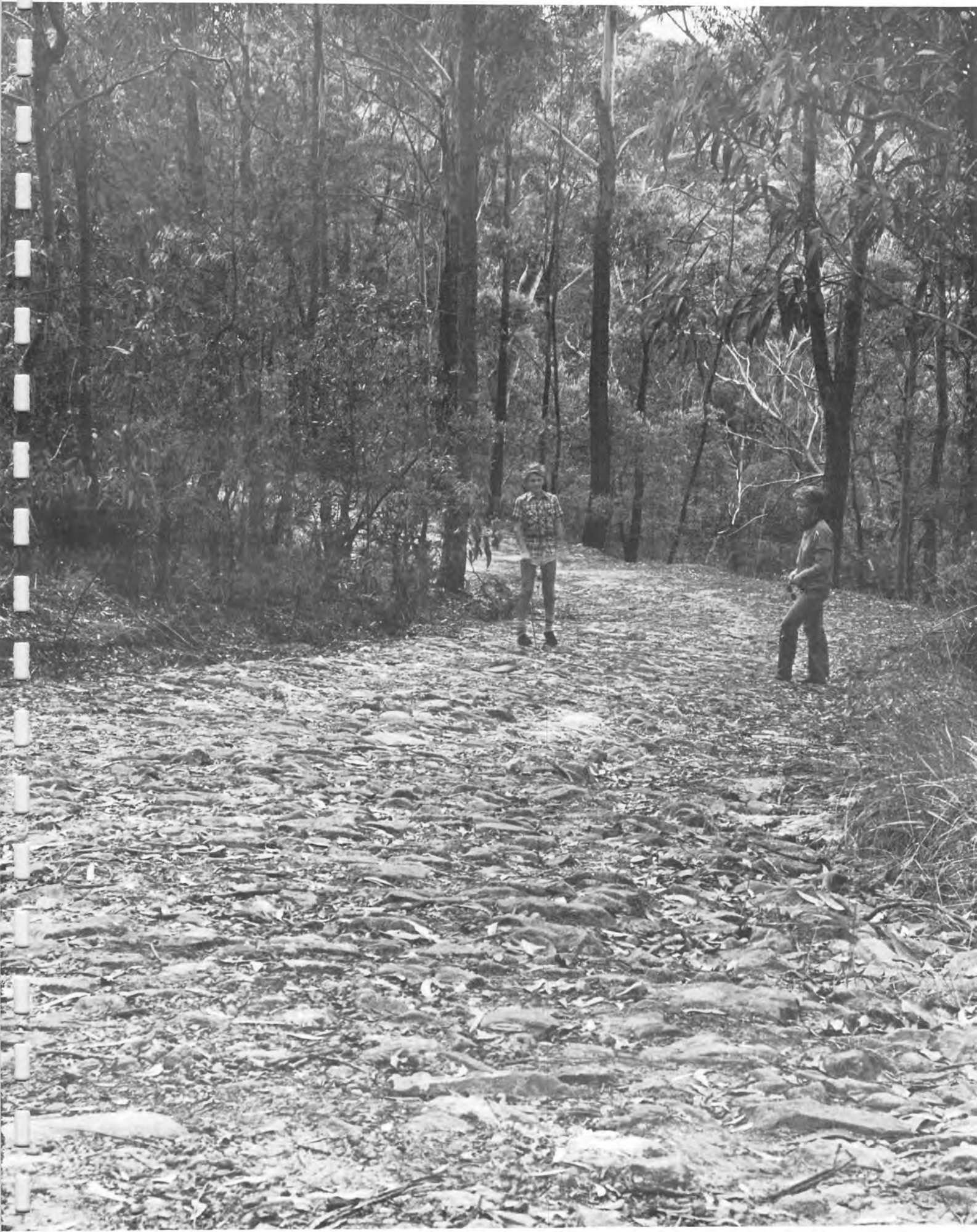
Old Road Built of Sandstone "Cobbles"
